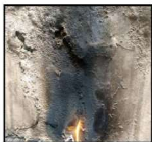
Fig. 4: First pattern formed on the vertical wall after diesel was spilled and then burned.
